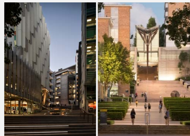
Public interface and front door | AUT SIR PAUL REEVES BUILDING (JASMAX) | UNSW KENSINGTON CAMPUS
