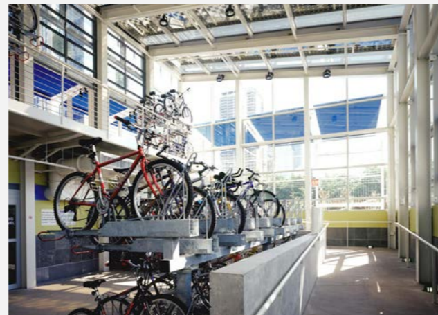
Secure bicycle storage, lockers, showers & bike repair areas provided to promote commuter bicycle transit into downtown Chicago | MCDONALD'S CYCLE CENTRE CHICAGO (MULLER&MULLER)
