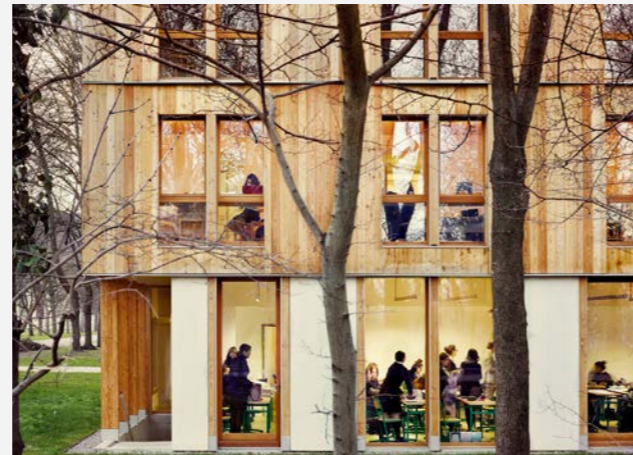
Timber-clad student dorms and educational centre set within a landscaped park for a boarding school in Paris | MAISON D'EDUCATION DE LA REGION D'HONNEUR (BELUS & HENOCQ ARCHITECTES)
